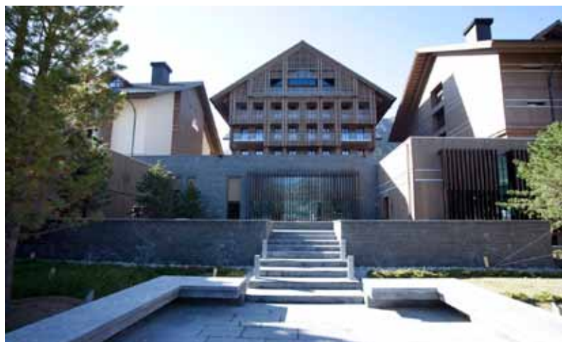
The four hotel buildings match the town’s aesthetic.
