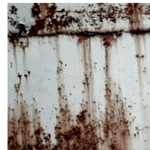
Protection from rust and corrosion
